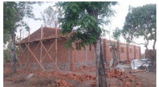
Liziyi church construction
